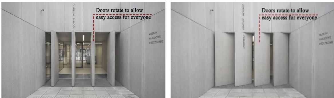
Figure 3-7: Entrance Source: KWK Promes Konieczny, 2015
