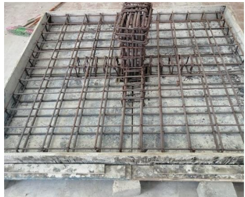
d) Distance between stirrups 70mm.
