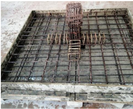
c) Distance between stirrups 50mm.
