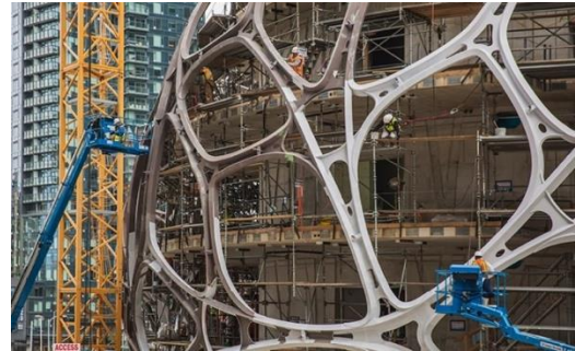
fig. 20 Fabrication and installation of the Catalan steel structure [34]
