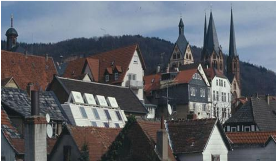
Figure 13: Perspective view showing the respectful Living room house with its surrounding historical context
