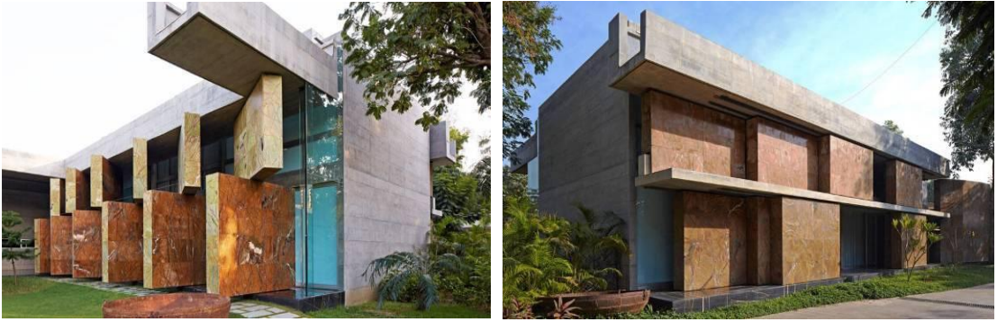
Figure 5: Massive stone walls rotate to bring natural light inside home Source: https://inhabitat.com/massive-stone-walls-rotate-to-bring-natural-light-inside-this-extraordinary-indian-home
